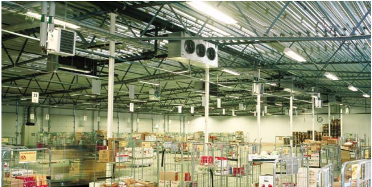
In a food store it is extremely important that the temperature is neither too high nor low. Fan heater SW is easy to control.
