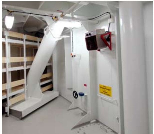
Vibrations onboard ships and offshore platforms can cause electronic equipment to malfunction. Elektra V fan heater has been designed to overcome these stresses.
