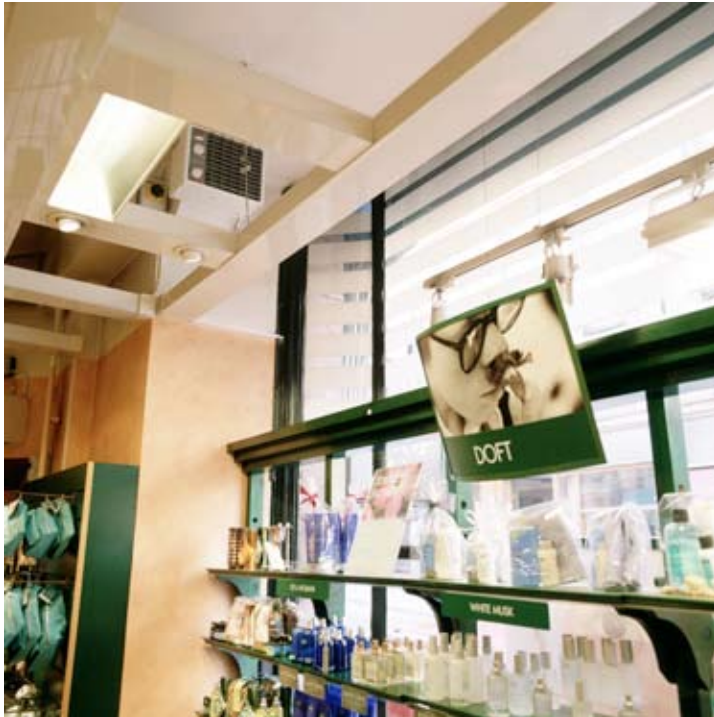
The Cat fan heater with mixing cabinet can easily solve problems in premises with negative pressure. Cold air is taken in from below and then heated before being released out into the premises.
